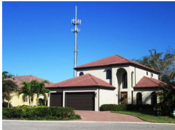
View of tower from front of house looking north
