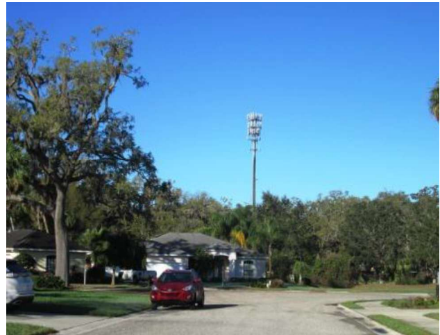
View of tower from front of property
