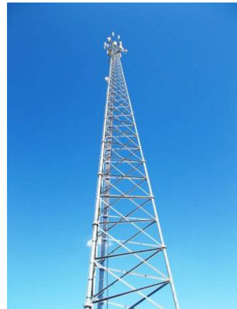
View of tower from the base compound
