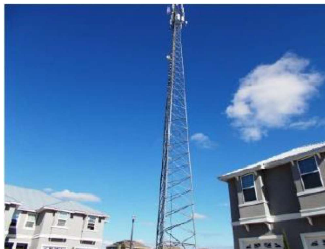
View of tower from adjoining apartments
