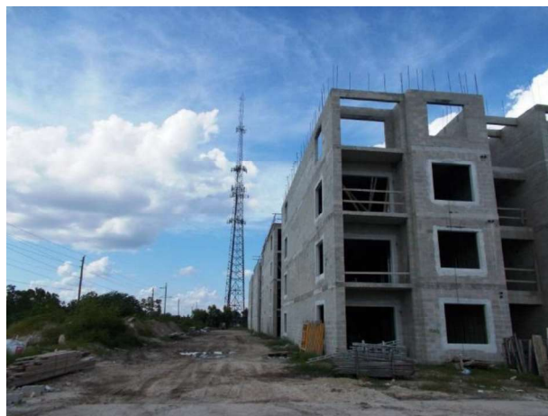
Azaela Park Rental Community under construction
