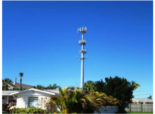
View of tower in front of 313 58 th Street
