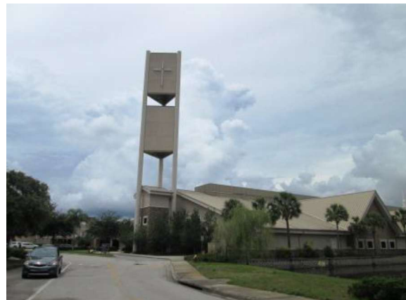
Street view of bell tower installation
