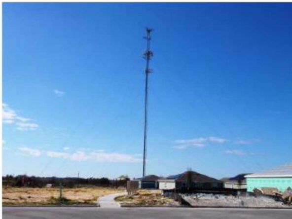
Street view of tower from Polk City Road
